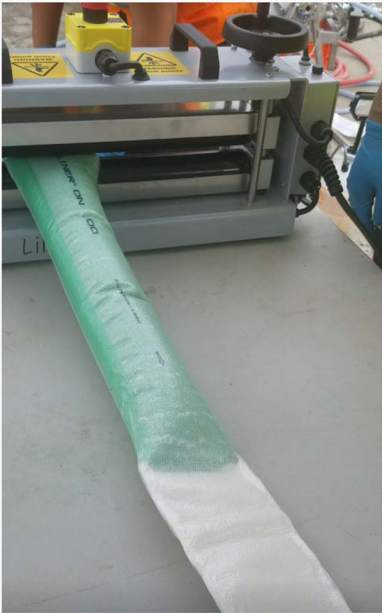
Wet-out liner before resin distribution and calibration
